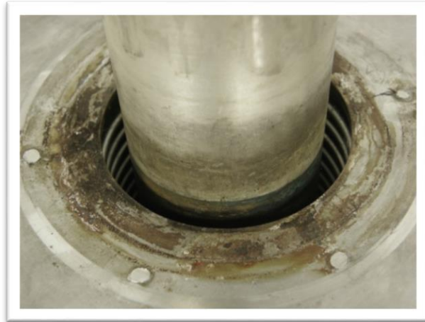
Image 1 - Saltwater corrosion.
